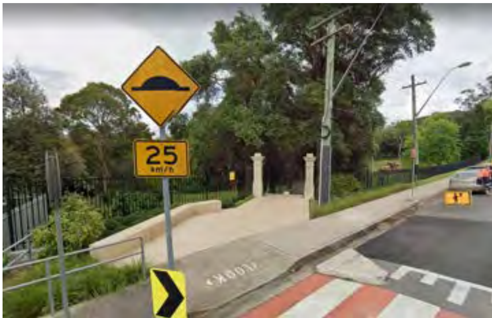
FIGURE 2. MAIN PEDESTRIAN ACCESS
