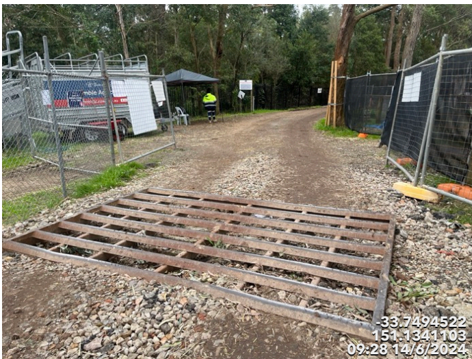
Photo 9 Rumble grid was installed
