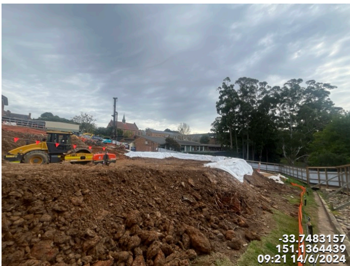
Photo 2 First layer of earth bund was create to collect surface water
