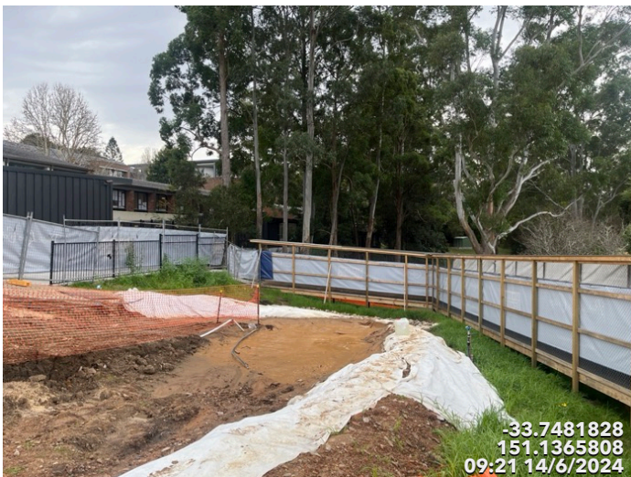
Photo 3. Lower bund was created and additional sediment control
