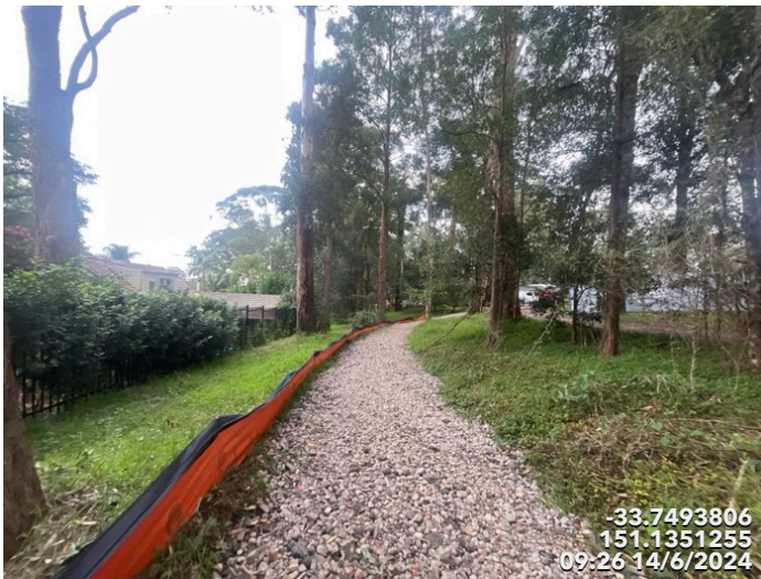
Photo 7 Sediment Fence and Pedestrian pathway was installed
