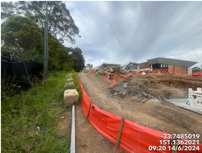
Photo 1 Sediment Fence was installed as per Blue book
